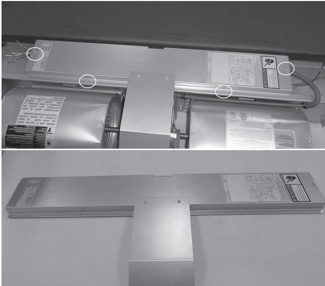
Fig. 6 - Control Box Cover Removal
