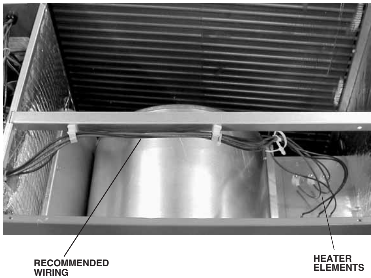
FIGURE 5 HEATER KIT INSTALLATION
